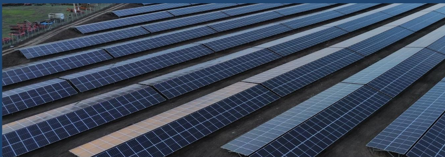
Premier Energy's 23 MW solar park development with a battery storage capacity of 10 MWh located in Nanov, Teleorman county, Romania.
